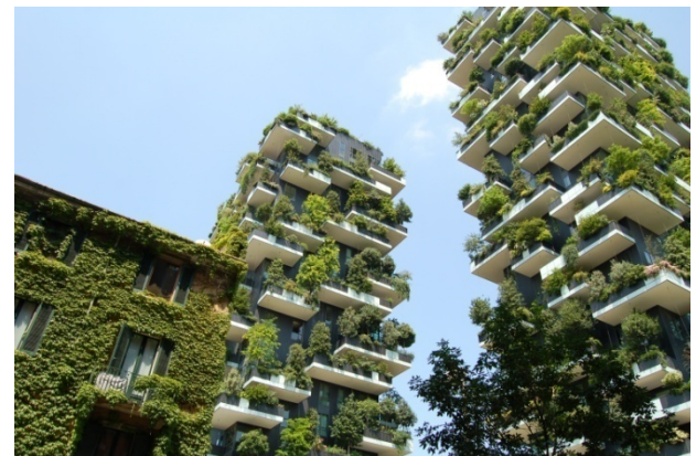
Figure 5: Bosco Verticale, Stefano Boeri & partners 2014. Detail of the facade.
